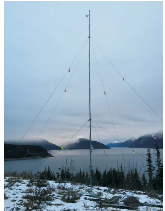
Met tower installation with Hero Data Logger in Haines, Alaska. Photo courtesy of Rich Stromberg of AEA.
